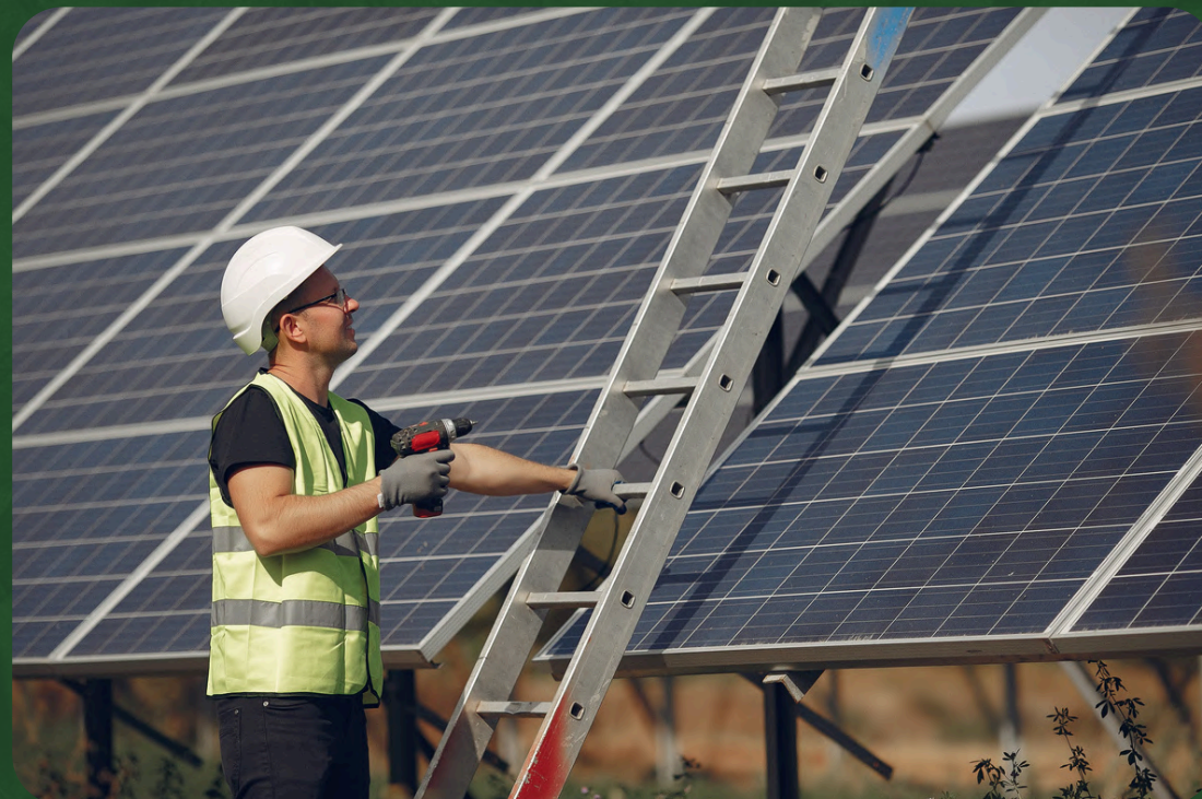
Maintenance and Care
